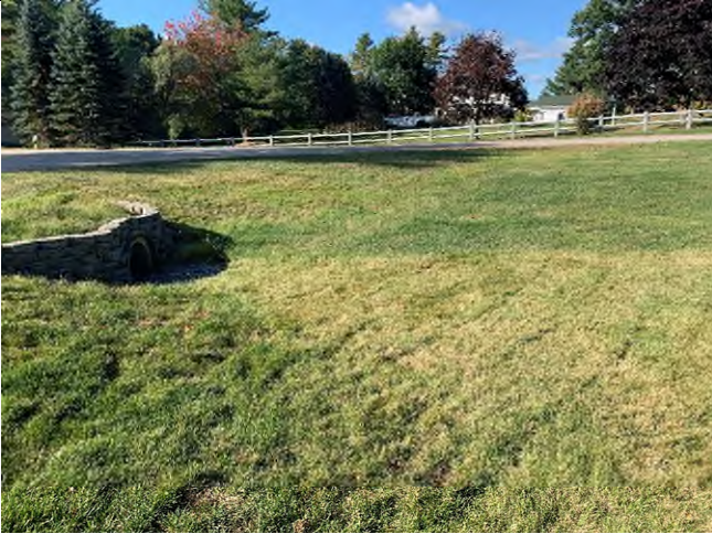
29 Gundalow - 1 (Drainage Area)
